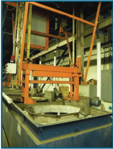
DIFCO engineers design, fabricate and install their own equipment, including this line dedicated to processing bulk parts.
